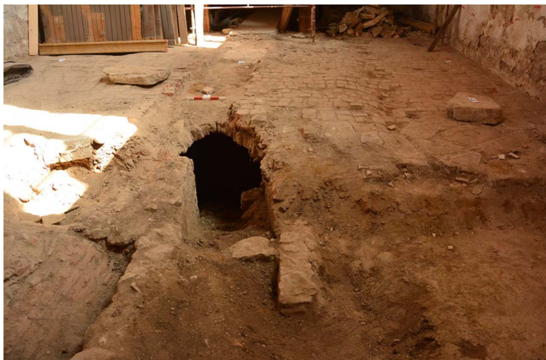
Fig. 1. Collapsed vault in the sanctuary of the Calvinist Church in Huedin (image from the MNIT Archive).
